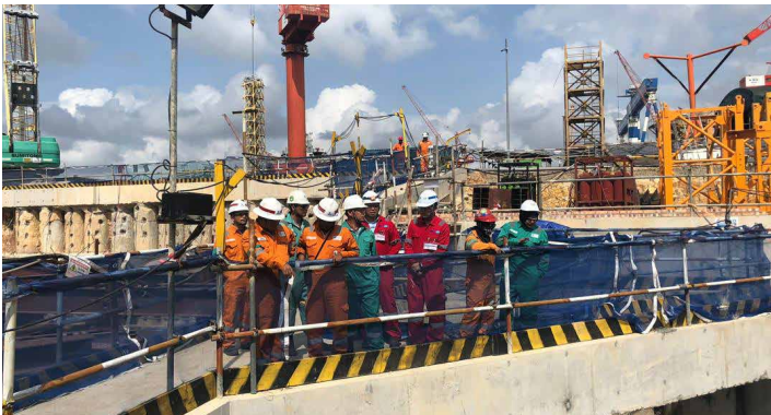
Site Inspection by the Department of Occupational Safety and Health of Malaysia
