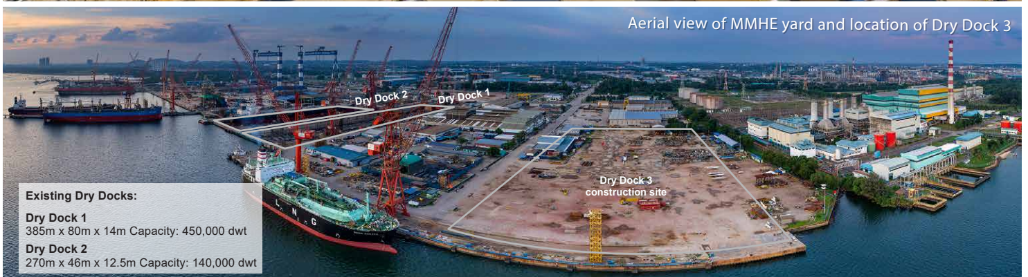
Aerial view of Dry Dock 3 construction site taken on 31st March 2019
