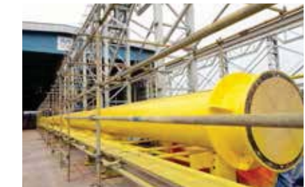
Kanowit Host Tie-in Brownfield (82 days) Client : PETRONAS Carigali Sdn Bhd
